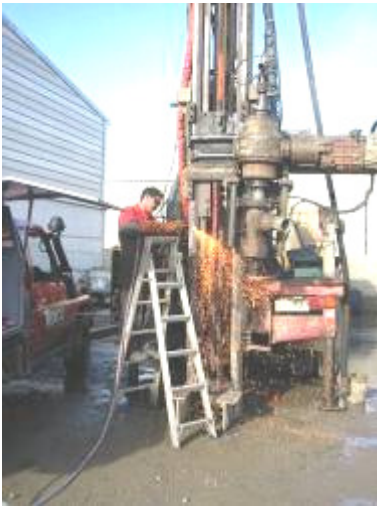
Dismantling the original unit.
